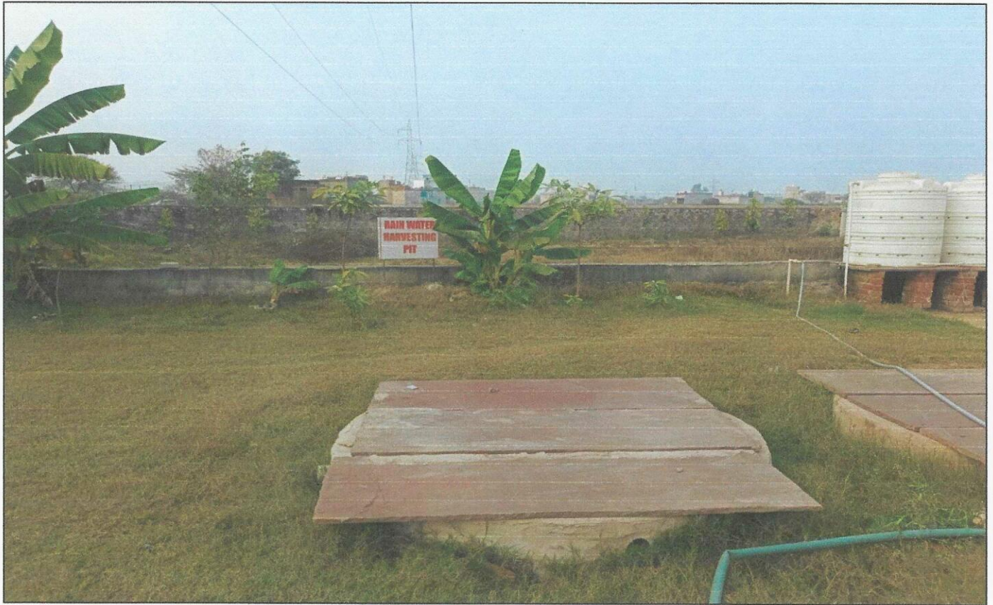
1 st RAIN WATER HARVESTING
