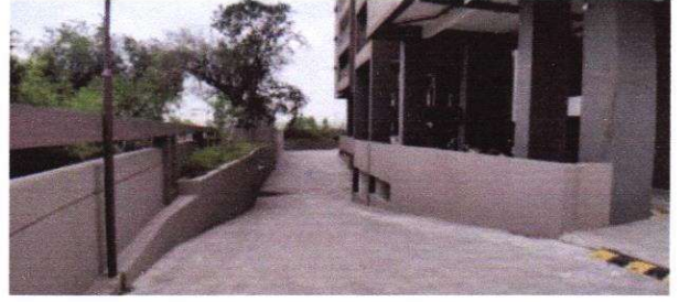
Ramp to Basement
