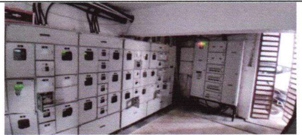
Electrical Panels of Flat Units
