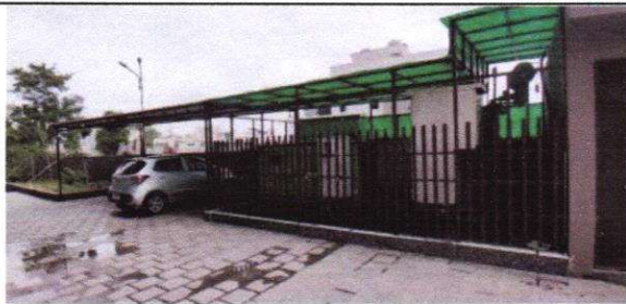
Transformer & Electrical Sub Station
