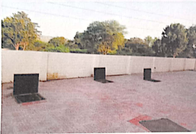
RAIN WATER HARVESTING
