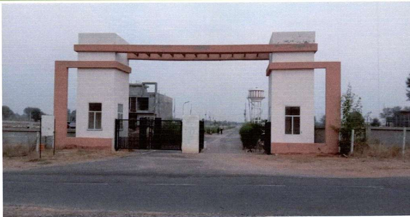
MAIN ENTRANCE OF THE SCHEME
